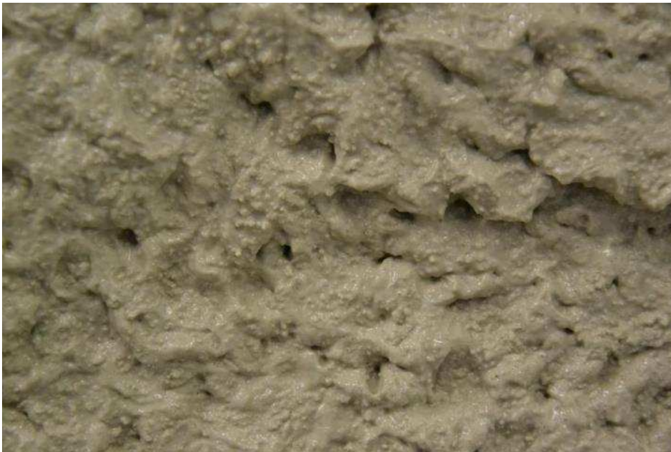
Close-up, fresh mortar
