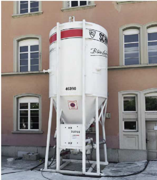
Delivery of the external render as dry mortar in a silo
