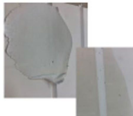
Application of the Patching filler on wall cracks
