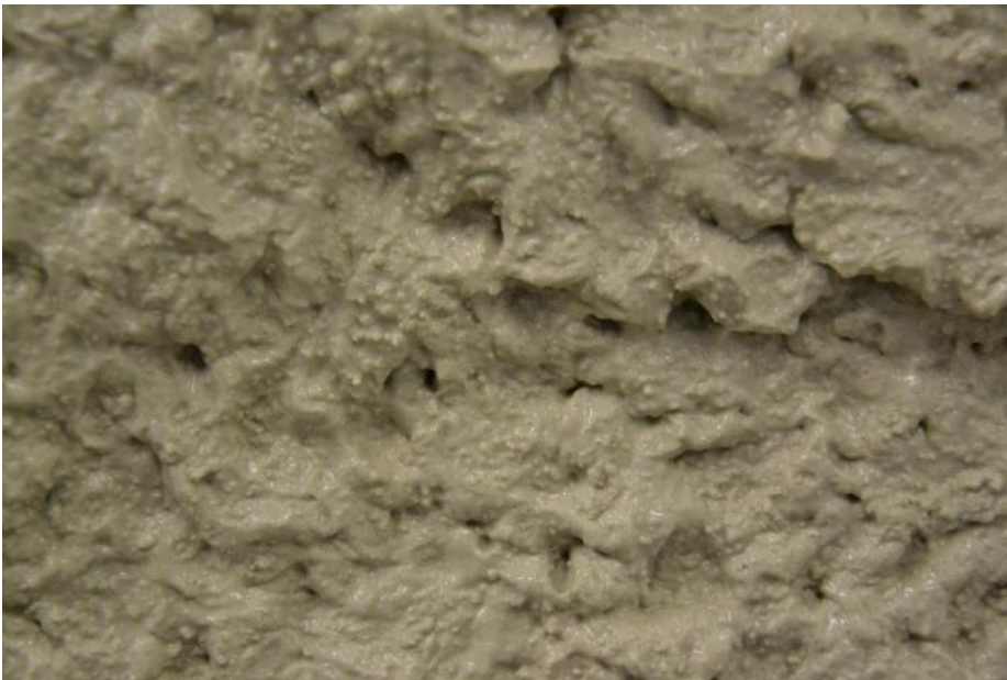
Close-up, fresh mortar
