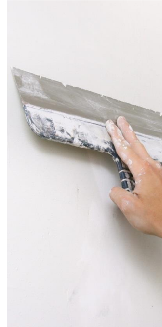
Thermal Coating Finishing
