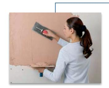
Insulating thermal coating finishing
